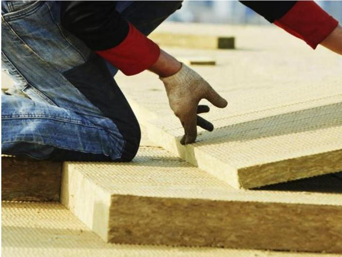
CCEWOOL® Stone Wool Board HD serves as an ideal substrate for mechanically fastened membrane systems, offering excellent soundproofing and thermal insulation performance. It can be used as the thermal base layer in soundproofing assemblies or combined with other roofing insulation materials to form the top layer of hybrid roof assemblies. To meet diverse application needs, CCEWOOL® Stone
