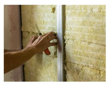
CCEWOOL® Stone Wool Board 40 is a high-performance stone wool insulation board designed for perimeter fire protection systems, floor and wall penetrations, construction joints, and other fire-related applications. The product is non-combustible and fire-resistant, ensuring that even when exposed to flames, it will not produce toxic smoke or contribute to flame spread, providing reliable fire
