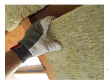
CCEWOOL® Stone Wool Sound Board is a high-performance Stone wool insulation product designed for interior partitions in wood and steel stud structures that require excellent fire protection and acoustic performance. This product can withstand high temperatures up to 2150°F (1177°C) and is non-combustible. Even when directly exposed to flames, it will not produce toxic smoke or contribute to the spread of
