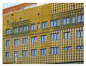
CCEWOOL® Stone Wool Board 40 is a high-performance stone wool insulation board designed for perimeter fire protection systems, floor and wall penetrations, construction joints, and other fire-related applications.
