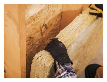
CCEWOOL® Stone Wool Batt is a high-performance semi-rigid stone wool insulation product specifically designed for new and renovated residential and commercial buildings. It is ideal for wall, ceiling, floor, and attic insulation systems in wood and steel-framed structures. This stone wool batt features unique flexible edges that can be easily compressed during installation, ensuring seamless filling of the
