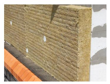
CCEWOOL® Stone Wool Board 45 is a high-performance semi-rigid stone wool insulation board specifically designed for concealed spaces in multi-unit residential buildings, providing exceptional fire and sound protection. With its superior fire resistance, ease of installation, and long-term stability, it is the ideal choice for ensuring fire safety in buildings, suitable for various protective needs in
