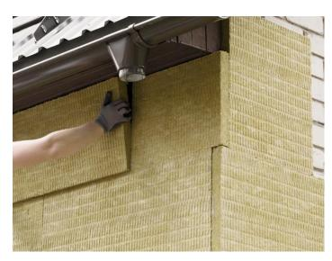
CCEWOOL® Stone Wool Board 55/65 is a medium-density Stone wool insulation product, specially designed for external and internal non-load-bearing steel firewalls, providing at least 1 hour of fire protection. CCEWOOL® Stone Wool Board 65 offers a fire rating of 1 hour, while CCEWOOL® Stone Wool Board 55 provides a 2-hour fire rating (measured from the interior side). These two products allow for more
