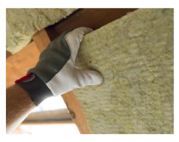
CCEWOOL® Rock Wool Sound Board is a high-performance Rock wool insulation product designed for interior partitions in wood and steel stud structures that require excellent fire protection and acoustic performance.
