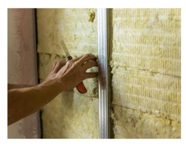
CCEWOOL® Rock Wool Board 40 is a high-performance Rock wool insulation board designed for perimeter fire protection systems, floor and wall penetrations, construction joints, and other fire-related applications.
