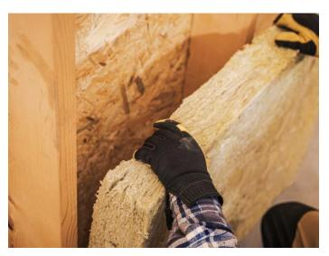
CCEWOOL® Rock Wool Batt is a high-performance semi-rigid Rock wool insulation product specifically designed for new and renovated residential and commercial buildings. It is ideal for wall, ceiling, floor, and attic insulation systems in wood and steel-framed structures. This Rock wool batt features unique flexible edges that can be easily compressed during installation, ensuring seamless filling of the
