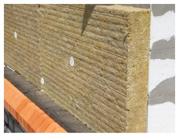
CCEWOOL® Rock Wool Board 45 is a high-performance semi-rigid Rock wool insulation board specifically designed for concealed spaces in multi-unit residential buildings, providing exceptional fire and sound protection. With its superior fire resistance, ease of installation, and long-term stability, it is the ideal choice for ensuring fire safety in buildings, suitable for various protective needs in
