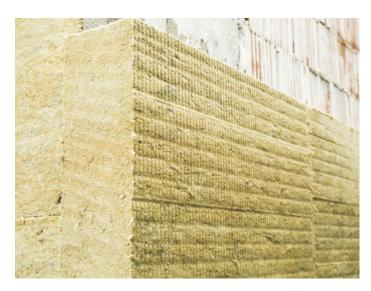
CCEWOOL® Rock Wool Board 110 is a high-density, rigid Rock wool insulation board with exceptional thermal, moisture-resistant, and vapor-permeable properties, designed for exterior continuous insulation applications. It is non-combustible, providing effective fire protection and moisture control, while offering superior thermal insulation to ensure high-performance wall systems. As an ideal
