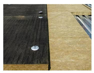
an ideal substrate for mechanically fastened membrane systems, offering excellent soundproofing and thermal insulation performance. It can be used as the thermal base layer in soundproofing assemblies or combined with other roofing insulation materials to form the top layer of hybrid roof assemblies. To meet diverse application needs, CCEWOOL® Rock
