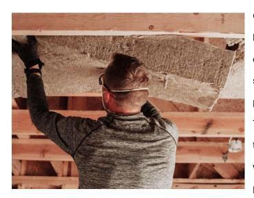
CCEWOOL® Rock Wool Sound Board is a high-performance rock wool insulation product designed for interior partitions in wood and steel stud structures that require excellent fire protection and acoustic performance. This product can withstand high temperatures up to 2150°F (1177°C) and is non-combustible. Even when directly exposed to flames, it will not produce toxic smoke or contribute to the spread of
