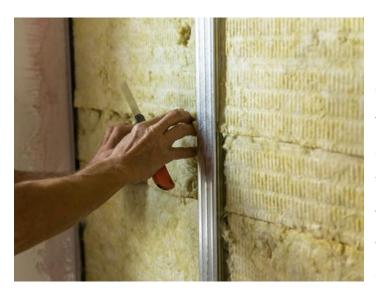
CCEWOOL® Rock Wool Board 40 is a high-performance stone wool insulation board designed for perimeter fire protection systems, floor and wall penetrations, construction joints, and other fire-related applications. The product is non-combustible and fire-resistant, ensuring that even when exposed to flames, it will not produce toxic smoke or contribute to flame spread, providing reliable fire
