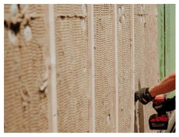
CCEWOOL® Rock Wool Board 45 is a high-performance semi-rigid stone wool insulation board specifically designed for concealed spaces in multi-unit residential buildings, providing exceptional fire and sound protection. With its superior fire resistance, ease of installation, and long-term stability, it is the ideal choice for ensuring fire safety in buildings, suitable for various protective needs in
