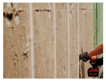
CCEWOOL® Rock Wool Board 45 is a high-performance semi-rigid stone wool insulation board specifically designed for concealed spaces in multi-unit residential buildings, providing exceptional fire and sound protection. With its superior fire resistance, ease of installation, and long-term stability, it is the ideal choice for ensuring fire safety in buildings, suitable for various protective needs in
