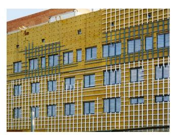
CCEWOOL® Rock Wool Board 40 is a high-performance stone wool insulation board designed for perimeter fire protection systems, floor and wall penetrations, construction joints, and other fire-related applications.
