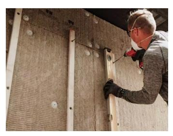
CCEWOOL® Rock Wool Board 80 is a high-performance rigid stone wool insulation board designed for exterior continuous insulation systems in both residential and commercial buildings. It offers exceptional thermal, fire-resistant, and acoustic performance.
