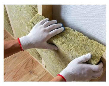
CCEWOOL® Rock Wool Batt is a high-performance semi-rigid stone wool insulation product specifically designed for new and renovated residential and commercial buildings. It is ideal for wall, ceiling, floor, and attic insulation systems in wood and steel-framed structures. This stone wool batt features unique flexible edges that can be easily compressed during installation, ensuring seamless filling of the
