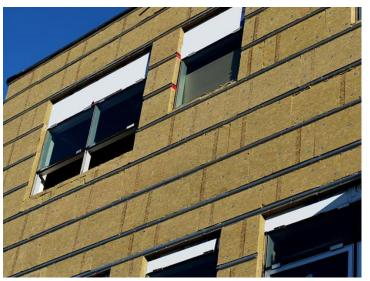
CCEWOOL® Curtain Wall Insulation Board is a high-performance semi-rigid stone wool insulation board designed for curtain wall systems. It offers outstanding fire protection and thermal performance. Its non-combustible properties ensure that it will not produce smoke or contribute to flame spread when exposed to fire, providing reliable safety for buildings.
