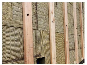
CCEWOOL® Rock Wool Board 110 is a high-density, rigid stone wool insulation board with exceptional thermal, moisture-resistant, and vapor-permeable properties, designed for exterior continuous insulation applications. It is non-combustible, providing effective fire protection and moisture control, while offering superior thermal insulation to ensure high-performance wall systems. As an ideal
