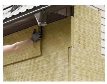
CCEWOOL® Rock Wool Board 55/65 is a medium-density rock wool insulation product, specially designed for external and internal non-load-bearing steel firewalls, providing at least 1 hour of fire protection. CCEWOOL® Rock Wool Board 65 offers a fire rating of 1 hour, while CCEWOOL® Rock Wool Board 55 provides a 2-hour fire rating (measured from the interior side). These two products allow for more flexible
