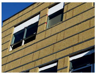
CCEWOOL® Curtain Wall Insulation Board is a high-performance semi-rigid stone wool insulation board designed for curtain wall systems. It offers outstanding fire protection and thermal performance. Its non-combustible properties ensure that it will not produce smoke or contribute to flame spread when exposed to fire, providing reliable safety for buildings.
