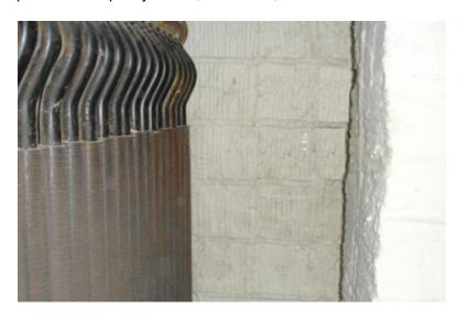
In the convection section of a primary reformer and, particularly, in the sidewalls and lower part of the end walls of a side-fired double-chamber primary reformer, there is a high gas flow velocity, requiring high resistance to erosion for the refractory lining. Therefore, high-strength refractory fiber castables or lightweight bricks are often used for
