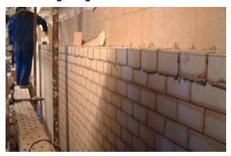
Considering the furnace temperature (usually about 1100℃) and a weak reducing atmosphere in the hydrogen production furnace as well as our years of design and construction experience and the fact that a large number of burners is generally distributed in the furnace at the top and the bottom and the sides of the wall, the lining material of
