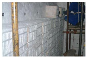
According to the characteristics of the anchoring structure of the fiber components, the furnace walls adopt "herringbone" or "angle iron" fiber components, which are arranged in the same direction along the folding direction. The fiber blankets of the same material between different rows are folded into a U shape to compensate for fiber shrinkage.
