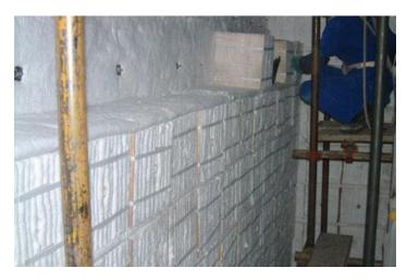
According to the characteristics of the anchoring structure of the fiber components, the furnace walls adopt "herringbone" or "angle iron" fiber components, which are arranged in the same direction along the folding direction. The fiber blankets of the same material between different rows are folded into a U shape to compensate for fiber
