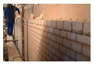
Considering the furnace temperature (usually about 700-800°C) and a weak reducing atmosphere in the decompression furnace as well as our years of design and construction experience and the fact that a large number of burners is generally distributed in the furnace at the top and the bottom and the sides of the wall, the lining material of decompression
