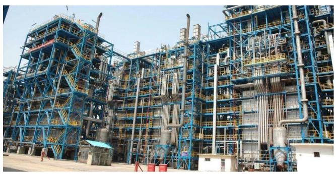
A cracking furnace is one of the key equipment in large-scale ethylene production units. It operates by using gaseous hydrocarbons (such as ethane, propane, and butane) and liquid hydrocarbons (such as light oil, diesel, and reduced-pressure diesel) as feedstock. These hydrocarbons undergo thermal cracking
