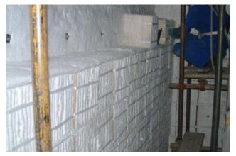
According to the characteristics of the anchoring structure of the fiber components, the furnace walls adopt "herringbone" or "angle iron" fiber components, which are arranged in the same direction along the folding direction. The fiber blankets of the same material between different rows are folded into a U shape to compensate for
