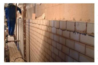
Considering the furnace temperature (usually about 700-800°C) and a weak reducing atmosphere in the atmospheric furnace as well as our years of design and construction experience and the fact that a large number of burners is generally distributed in the furnace at the top and the bottom and the sides of the wall, the lining
