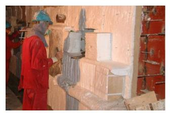
with two layers of CCEWOOL ceramic fiber blankets, and then stacked with the fiber components of a herringbone or angle iron anchor structure. The top of the furnace is tiled with two layers of CCEWOOL ceramic fiber and then stacked with the fiber components in the form of a single-hole hanging anchor structure.
