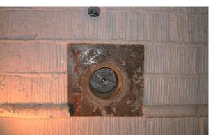
It adopts a layered-module composite lining structure with CCEWOOL 1260 ceramic fiber blankets for the back lining and CCEWOOL1430 zirconium-containing ceramic fiber modules for the hot surface. The ceramic fiber modules are arranged like "a battalion of soldiers", and the interlayer compensation blanket uses CCEWOOL1430 zirconium-containing ceramic fiber blanket, fixed by U-shaped heat-resistant steel nails.
