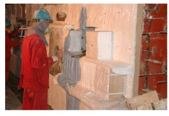
Considering the shape and structure of the heat treatment furnace, the furnace door and the bottom of the furnace door should be made of CCEWOOL fiber castable, and the rest of the furnace walls can be tiled with two layers of CCEWOOL ceramic fiber blankets, and then stacked with the fiber components of a herringbone or angle iron anchor
