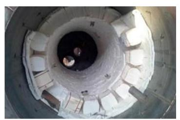
Performance comparison between the current structure of the steel (iron) ladle dryer and the original structure: It is recommended to use a tiled composite structure of CCEWOOL ceramic fiber blankets + CCEWOOL ceramic fiber modules with pickaxe.
