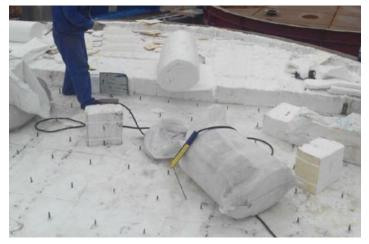
ceramic fiber modules with pickaxe is anchoring.
