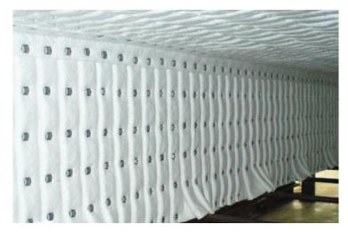
The shape of the heat exchange chamber is mostly square. When lining the side walls and end walls with ceramic fiber, the composite structure of tiled-laying and fiber prefabricated components is often adopted, in which the stacking layer of fiber components can be fixed with angle iron anchors.
